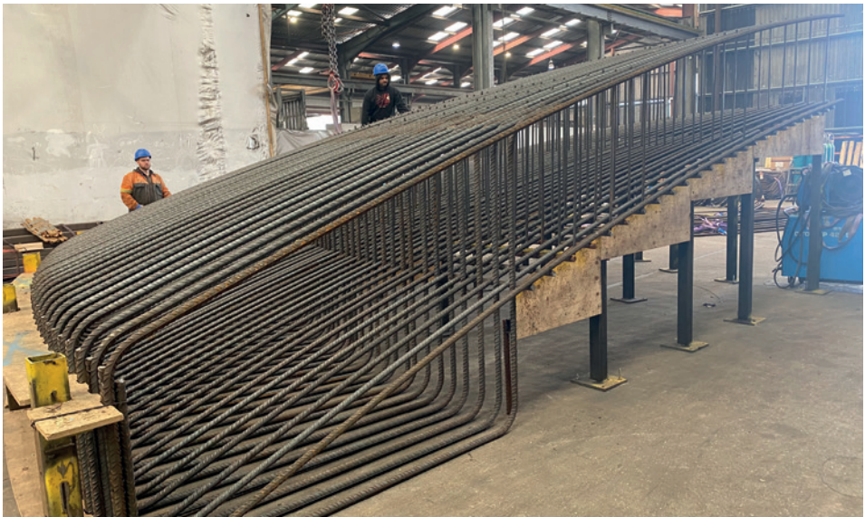
Figure 5. Early fabricator involvement ensures that the full benefits prefabrication can be realised
