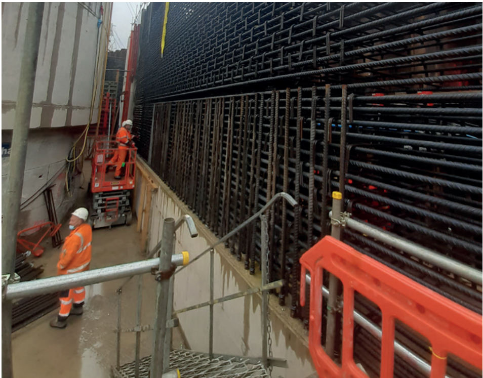
Figure 1. Early involvement facilitates the use of digital technology to redesign or even design out rebar thereby saving both construction time and money
